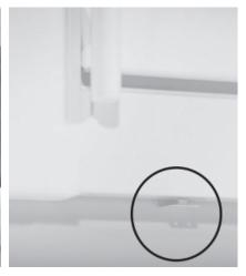
Using a credit card as a guide, slot a bracket into the corner of each rubber seal on the window.
