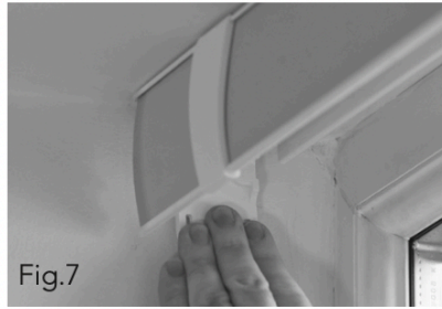
Fit the cassette back into the recess ensuring it is a snug fit and fold the lever brackets down to secure the blind. (Fig.6 & 7)
